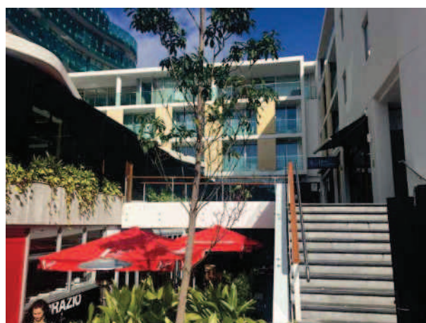
PICTURE 10 – RESIDENTIAL ABOVE RETAIL: HALL STREET, BONDI
